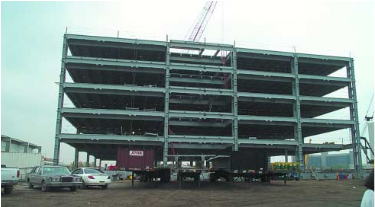
Erection of steel frames with precast deck in progress.
