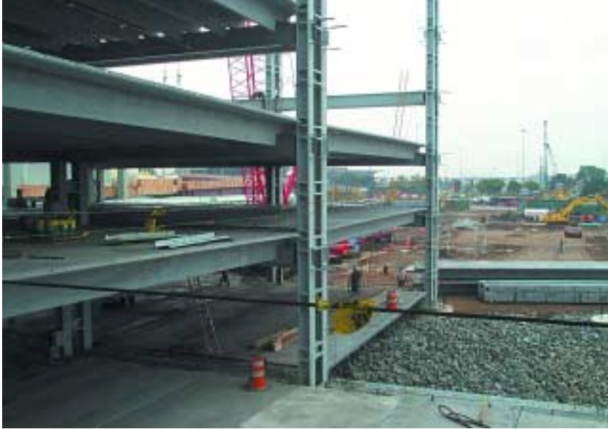
Erection of steel frames for Green Garage.
