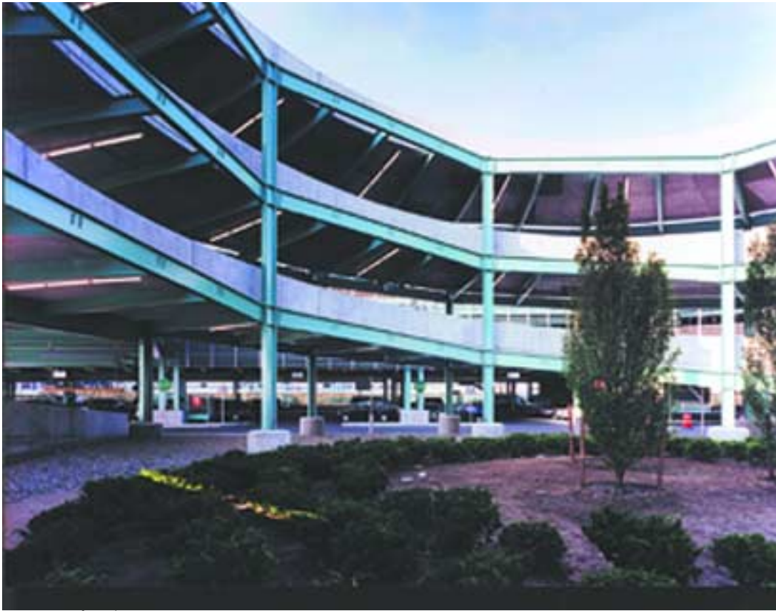
View of parking structure ramps.
