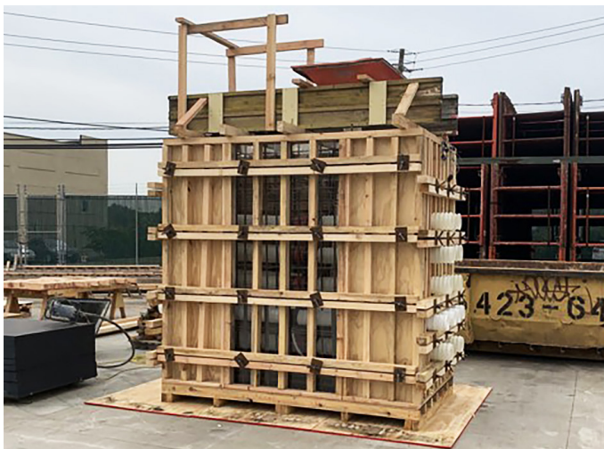
Fig. 11—PT girder mockup
