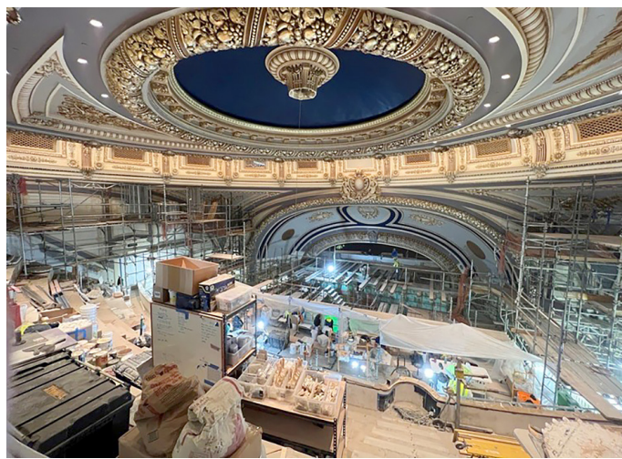
Fig. 2—Palace Theatre renovation
