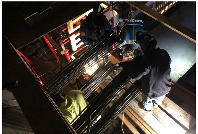
Fig. 7—Jacking operations
