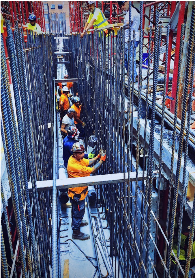
Fig. 14—PT girder construction
